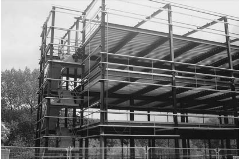
Fig. 22.1 Steel-framed office building under construction.
