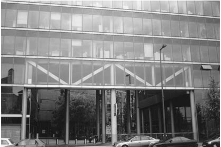
Fig. 12.5 Truss in façade, Sony Centre, Berlin.
