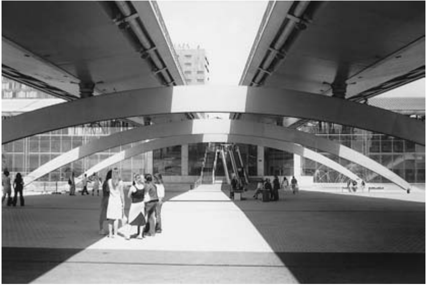
Fig. 17.4 Concrete arches supporting elevated roadway, Lille, France.
