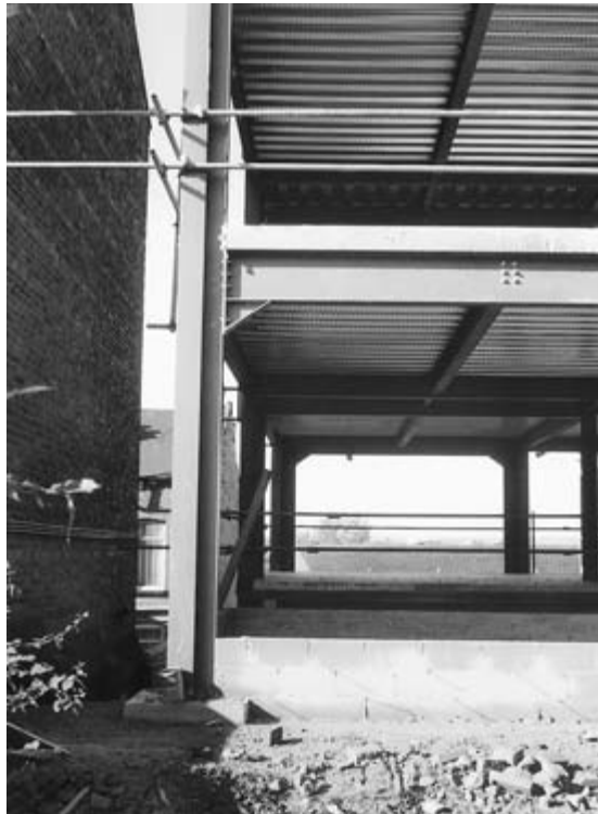
Fig. 9.2 Steel-framed building under construction.
